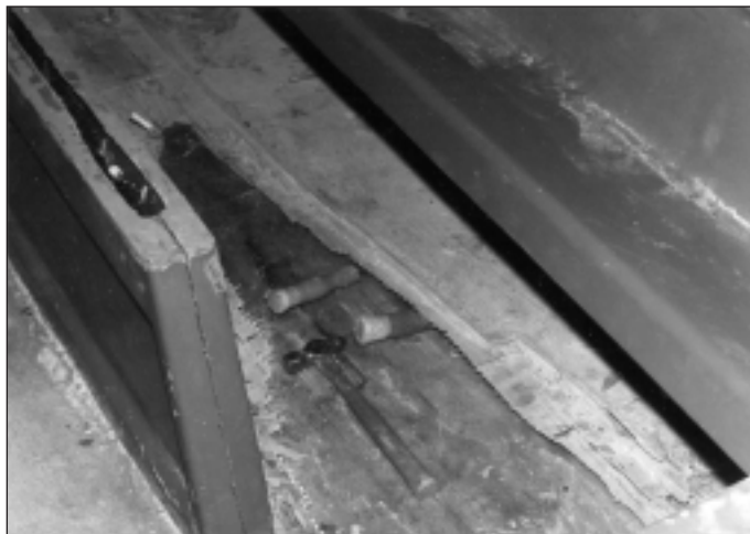
The original layer of balsawood being chiseled away.
